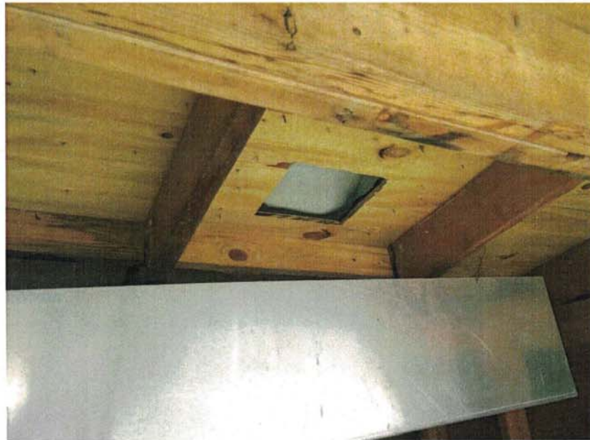
Photo No. 1 Interior of Deck at 35 mph
