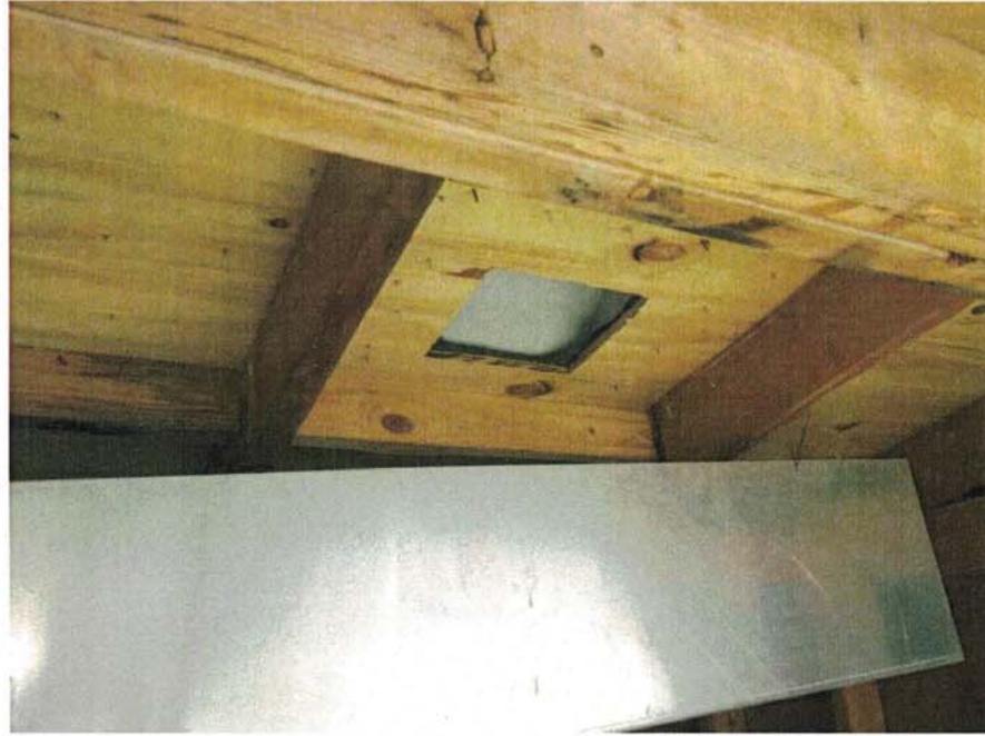
Photo No. 7 Interior of Deck at 110 mph
